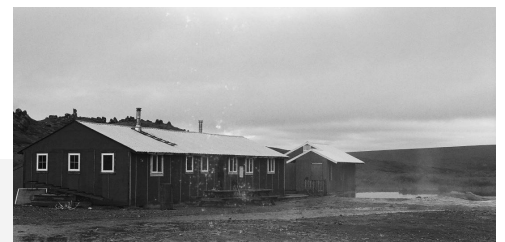
The Serpentine Hot Springs Bunkhouse
