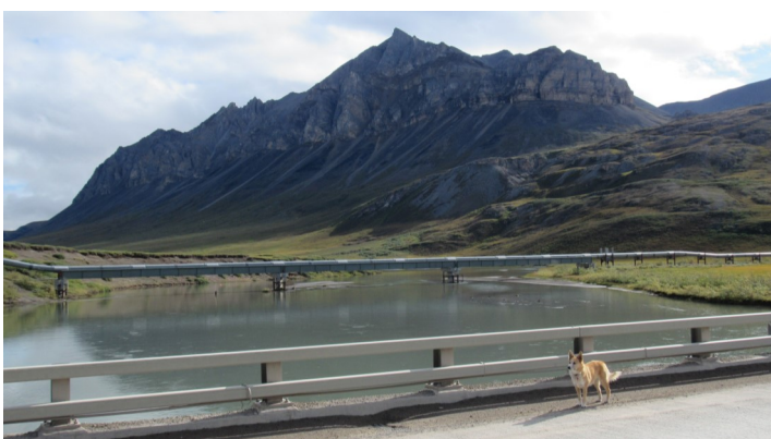
Crossing the Atigun River. Photo looks east.
