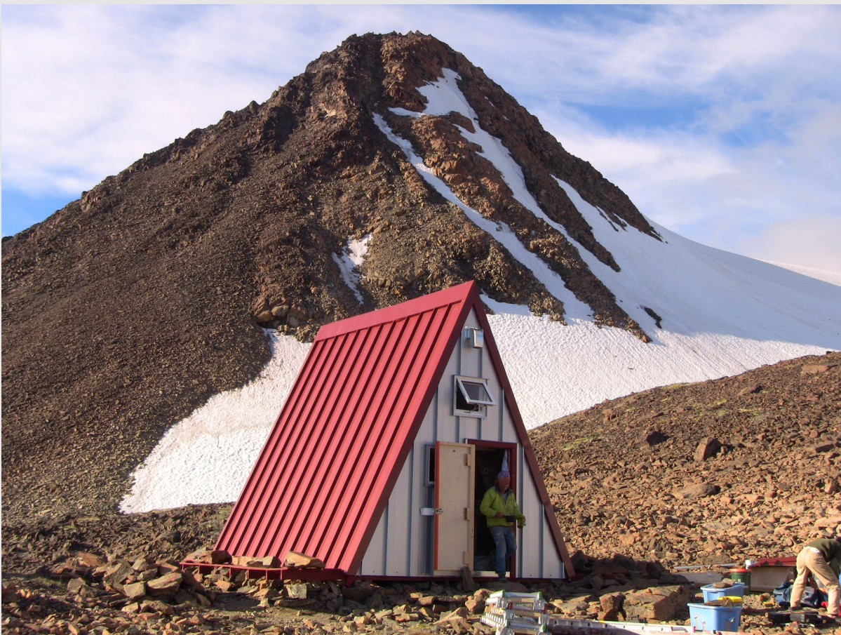
Stan Olsen exits the south side of the finished hut.
